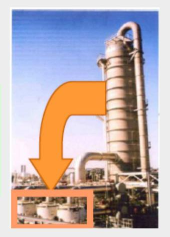
Conventional fixed bed reactor vs 40 times intensified reactor. (Source: Dow Chemical, proceso HOCI)
